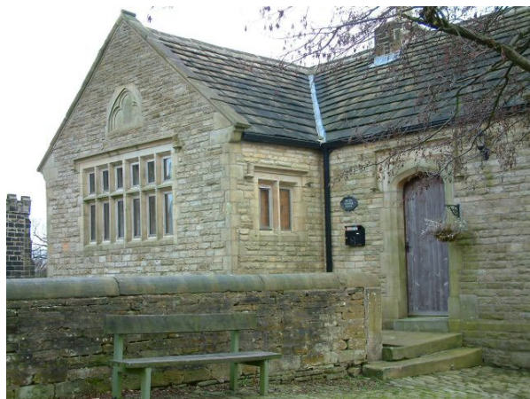
Figure 8: Mottram Old Grammar School, possibly Mottram Green School
