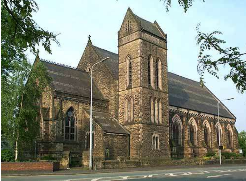
St Paul's Church, Coppenhall, Crewe 2
