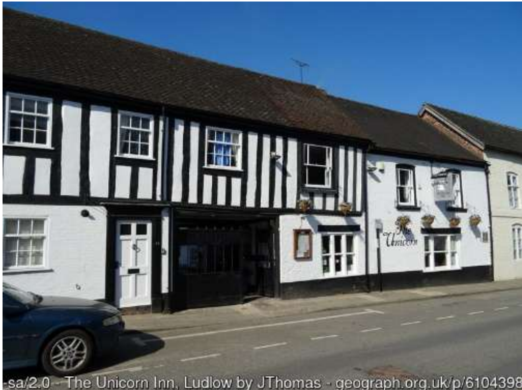
65 Lower Corve Street (the white door to the left of the picture) 8
