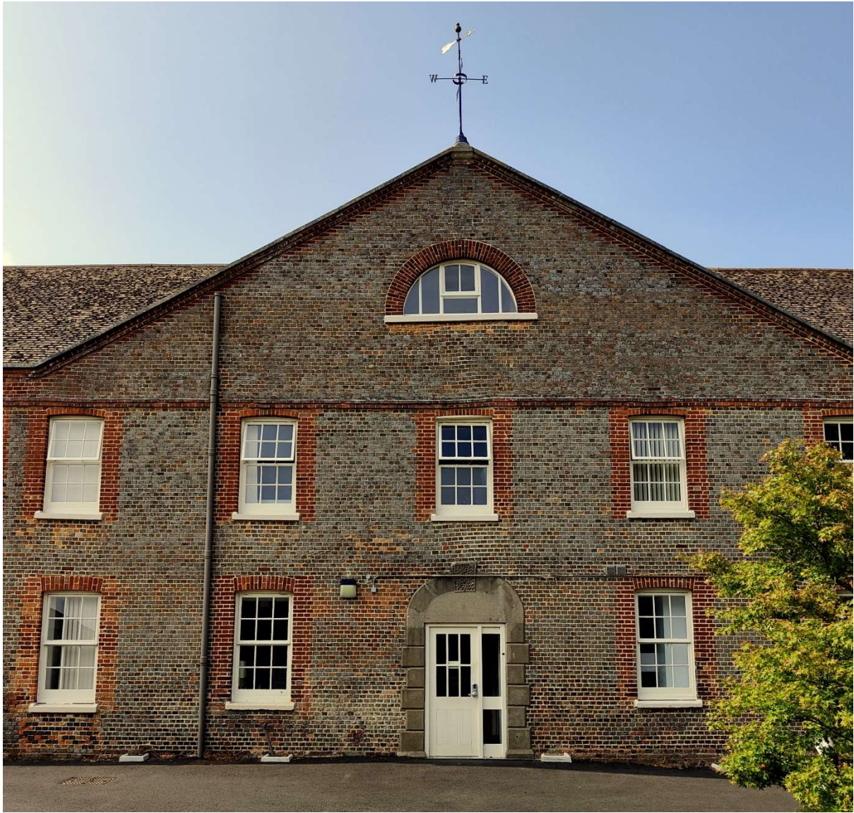
The House of Industry entrance, today part of St. Mary's hospital in Newport
