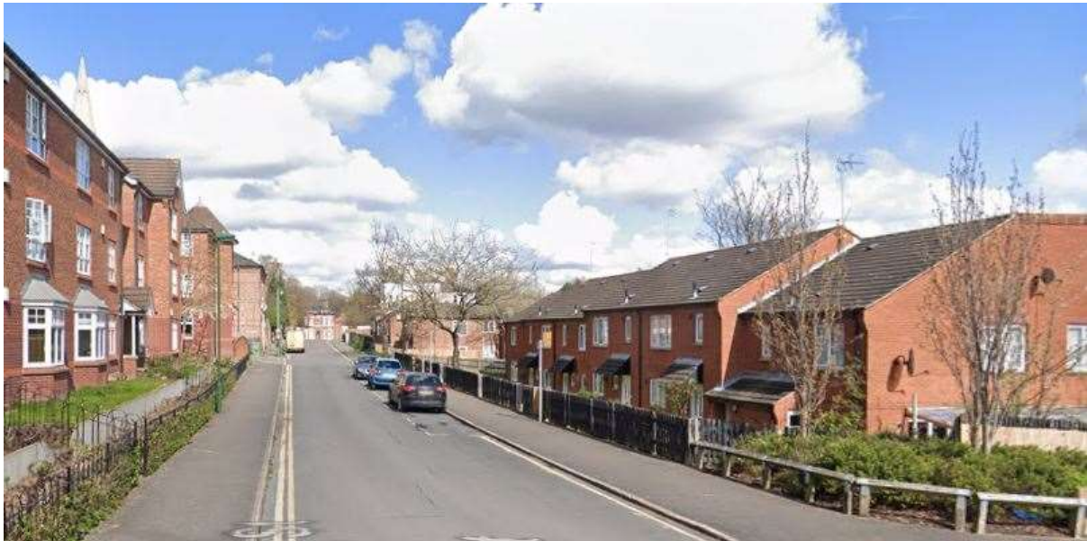
Raleigh Street, Nottingham, looking north-east towards All Saints' Church © Google Streetview
