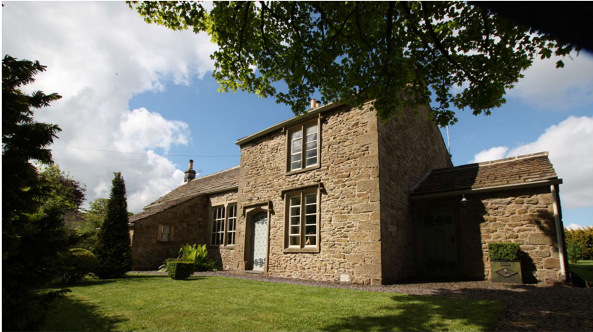
The former Tosside School Building Courtesy of MSW Hewetsons
